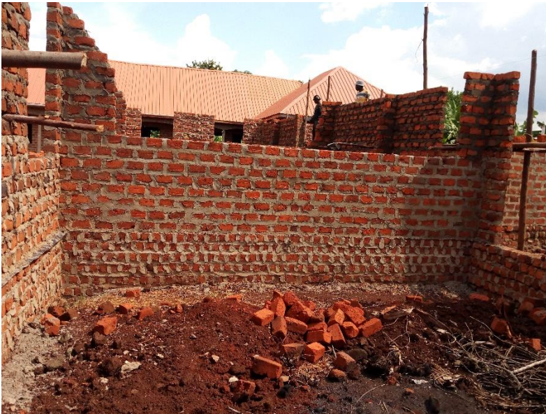
Stretching the inside walls that connect from the Top Classroom through the corridor
