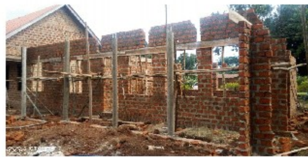
Nursery school in the construction phase
