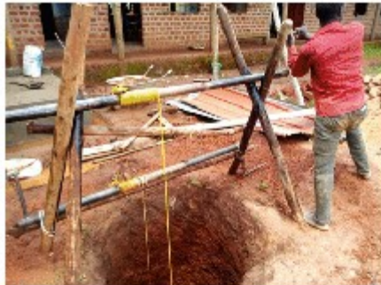
Drilling a well for water supply
